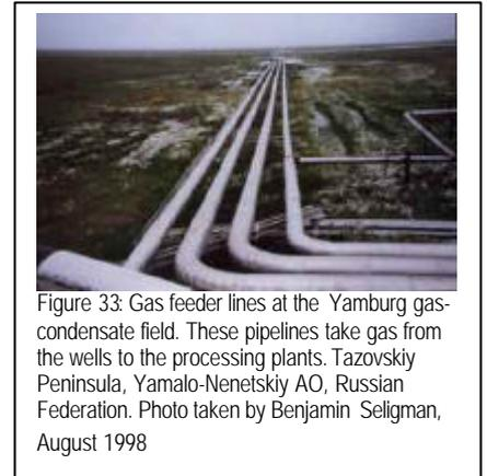
Figure 33: Gas feeder lines at the Yamburg gas-condensate field. These pipelines take gas from the wells to the processing plants. Tazovskiy Peninsula, Yamalo-Nenetskiy AO, Russian Federation. Photo taken by Benjamin Seligman, August 1998
